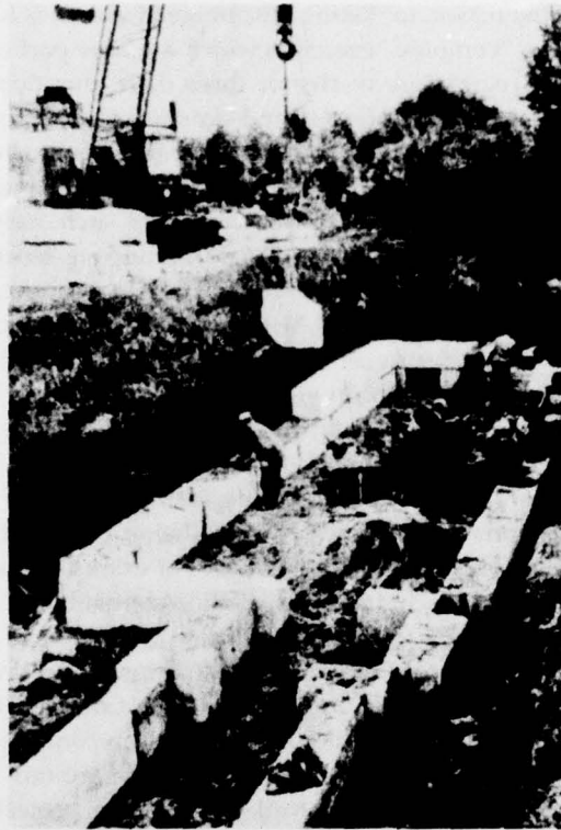
Hasty Shelter Under Construction
